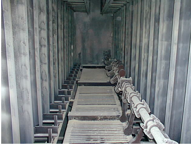
Fig. 2. Inner part of the ESP.
